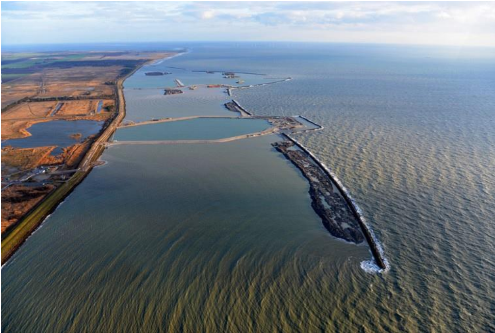
Fehmarn Belt Fixed Link working harbour under construction. January 2021
